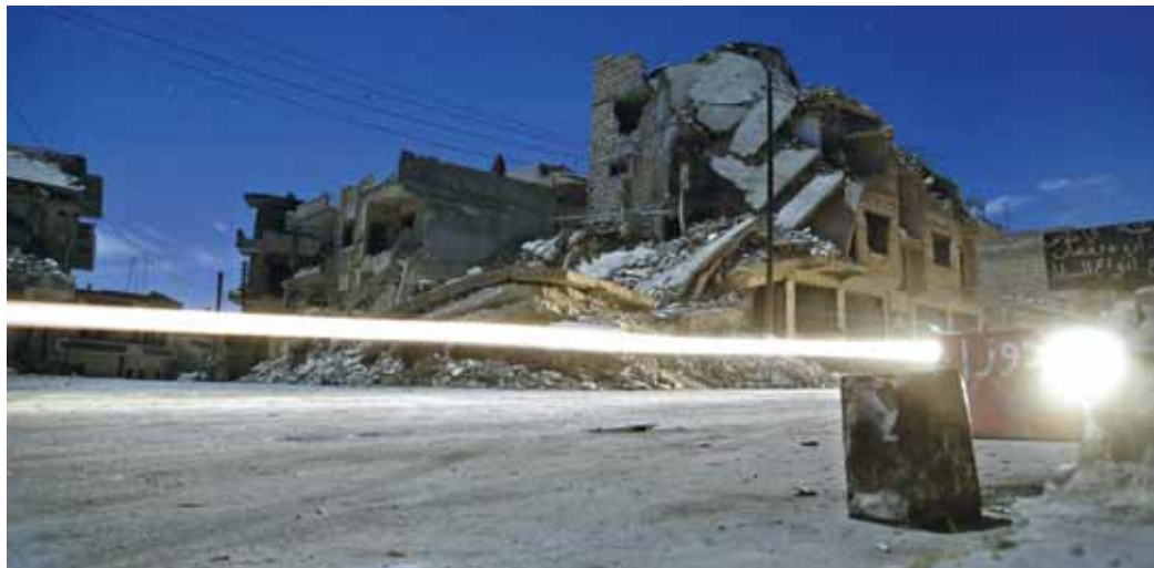
Damaged buildings are pictured at night in the rebel-controlled area of Maaret al-Numan town in Idlib province of Syria yesterday.
