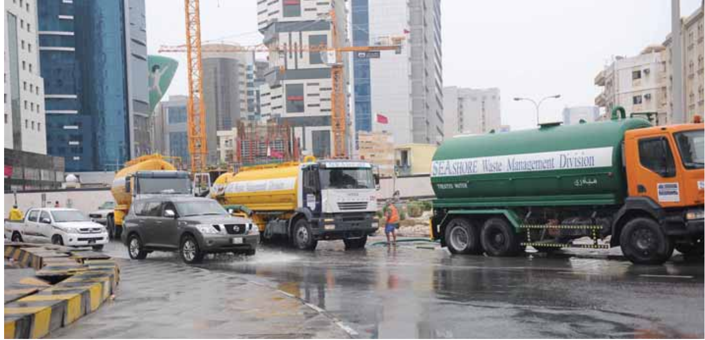
Suction trucks clearing the water at a roundabout.
