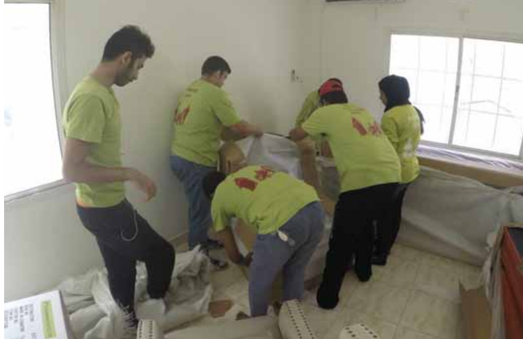
The renovation in progress.
